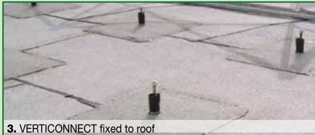
3. VERTICONNECT fixed to roof
