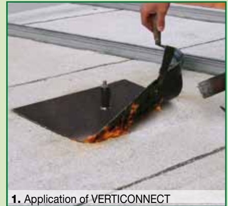
1. Application of VERTICONNECT
